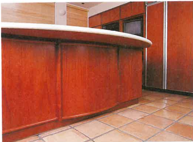
Figure 34-4. Large radius dry bend using 1/4" MDF panel with mahogany face veneers. The top and bottom half-round molding were steam bent and glued to the assembly. ( Chuck Davis Cabinets )
