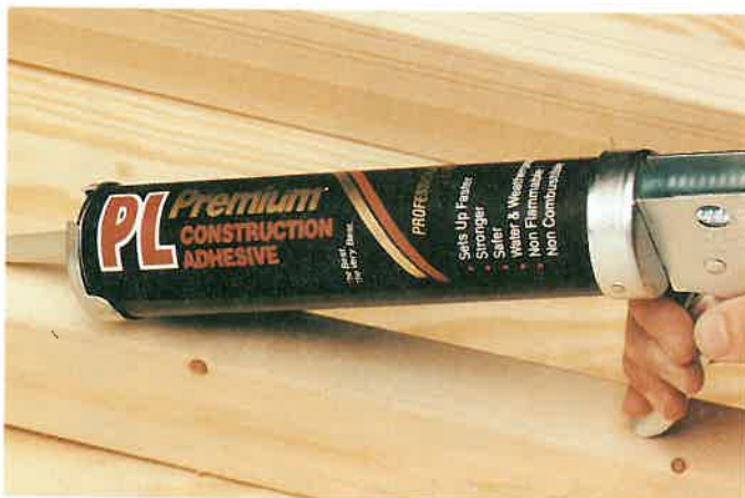
Figure 32-5. Construction adhesive is easily applied with a caulking gun. (Chemrex, Inc.)
