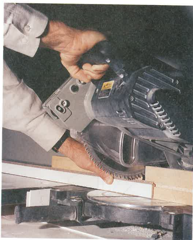
Figure 36-11. Trim the Perma-Edge® moldings about 1" (25.4 mm) longer than required. Note the groove in the temporary fence that is attached to the power miter saw. ( Wilsonart International )
